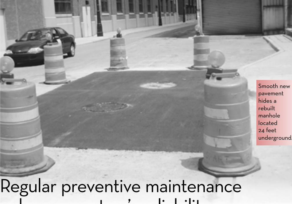
Smooth new pavement hides a rebuilt manhole located 24 feet underground.
