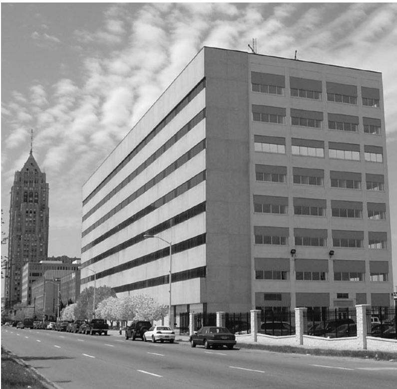
A steam trap survey was part of the restoration and improvement of 7310 Woodward.
