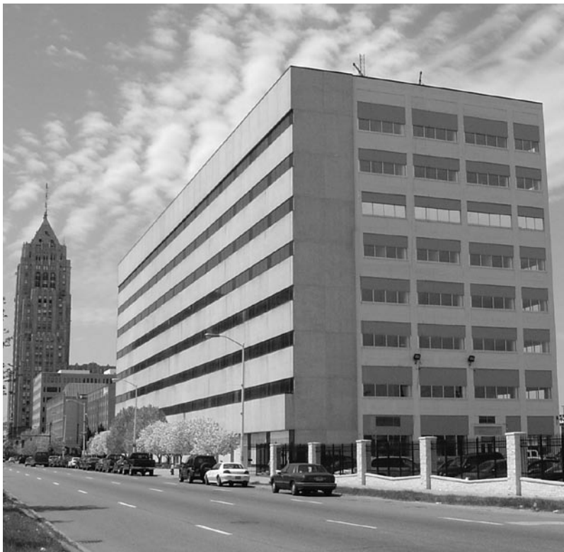
A steam trap survey was part of the restoration and improvement of 7310 Woodward.
